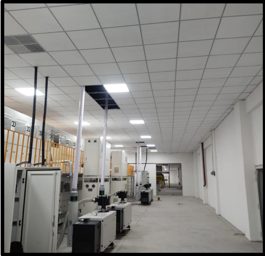
Duct covering and Planks
