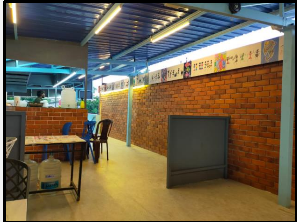
Back lining done with V Next Boards
