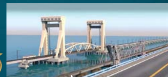
Most corrosive zone in the Indian peninsula and the crucial rail bridge at Pamban is being protected with Berger's Epilux 45 ZNPH (Anti-corrosive primer) and top coated with Berger Acrylic Poly Siloxane to give excellent colour and gloss retention. It's a pride of Berger for being the only choice supplier for protecting the entire 4,700 MT of steel used in the construction of this iconic sea bridge of INDIA.
