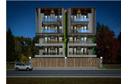
The Estate Apartments
