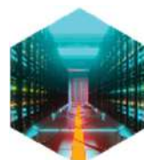
Telecom & Data Centers
