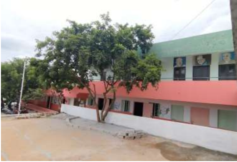
Renovation of classrooms, Uttarahalli - CKP
