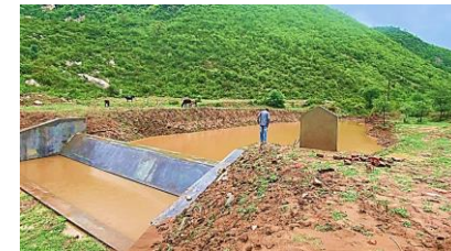
Water Conservation Project
