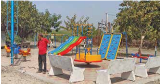
Installation of playing equipment for children at Dahej
