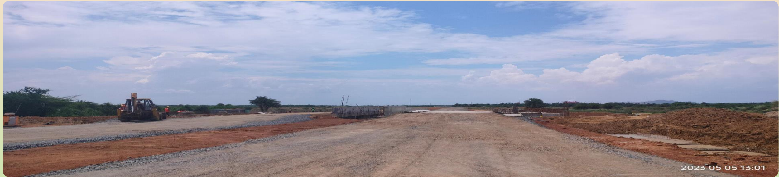
TSSEL- Access road & bridge over water body
