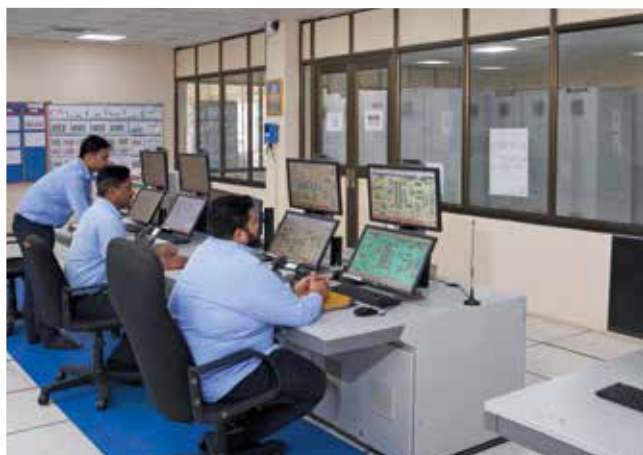
Main control room, Dahej Plant
