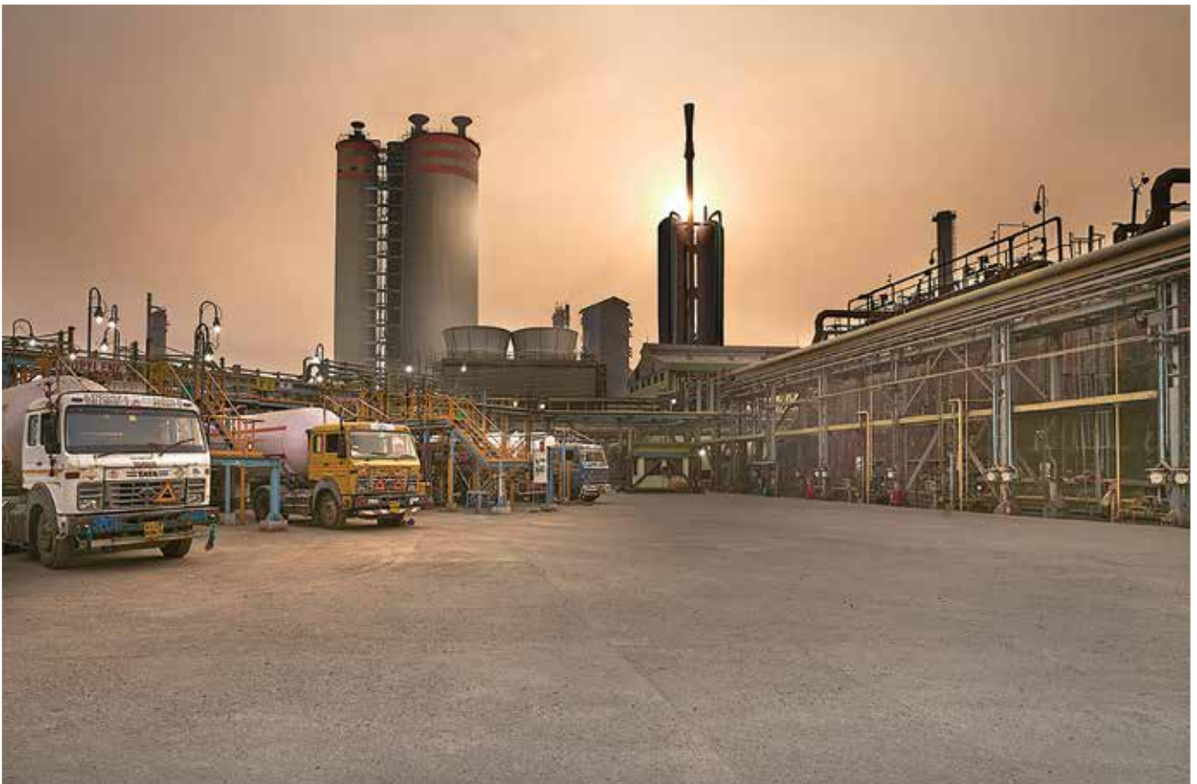
Sunset view of the K-1 plant taken from Propylene unloading area, with Prilling Tower and Nitric Acid Plants seen in the background
