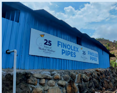
Renovation of a cow shed in Pune
