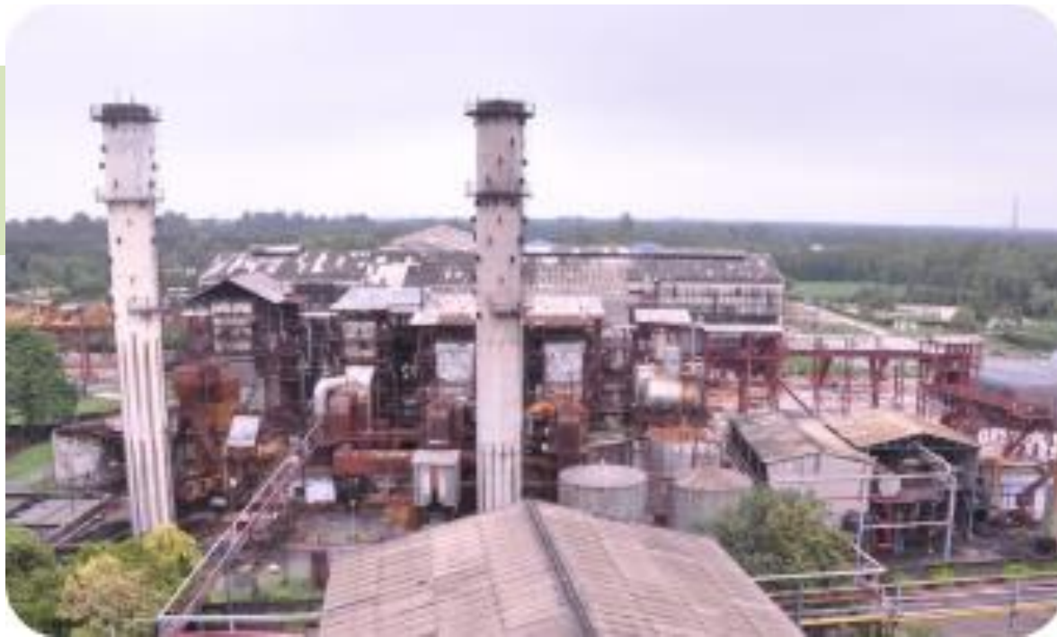
Sugar plant overview
