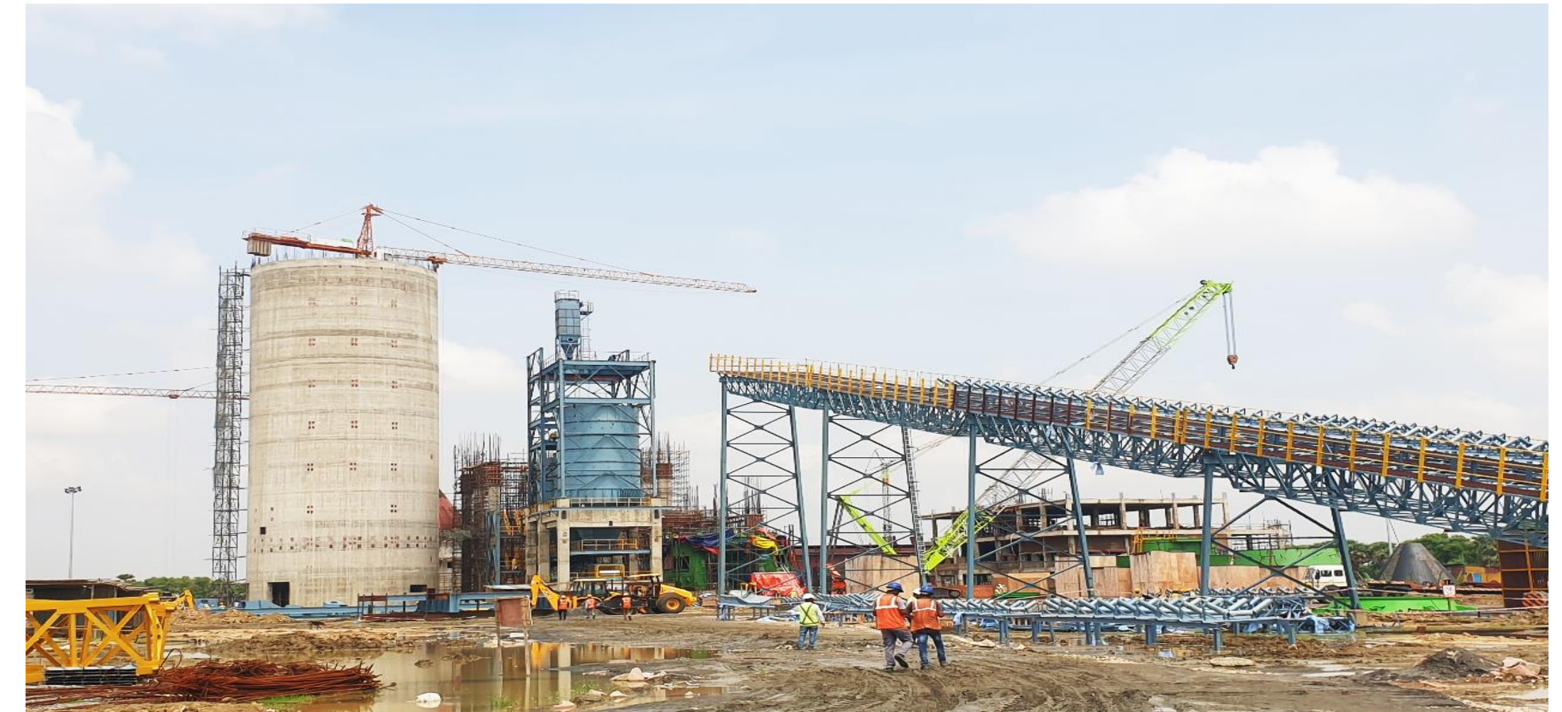
Belt Conveyor & Fly Ash Silo
