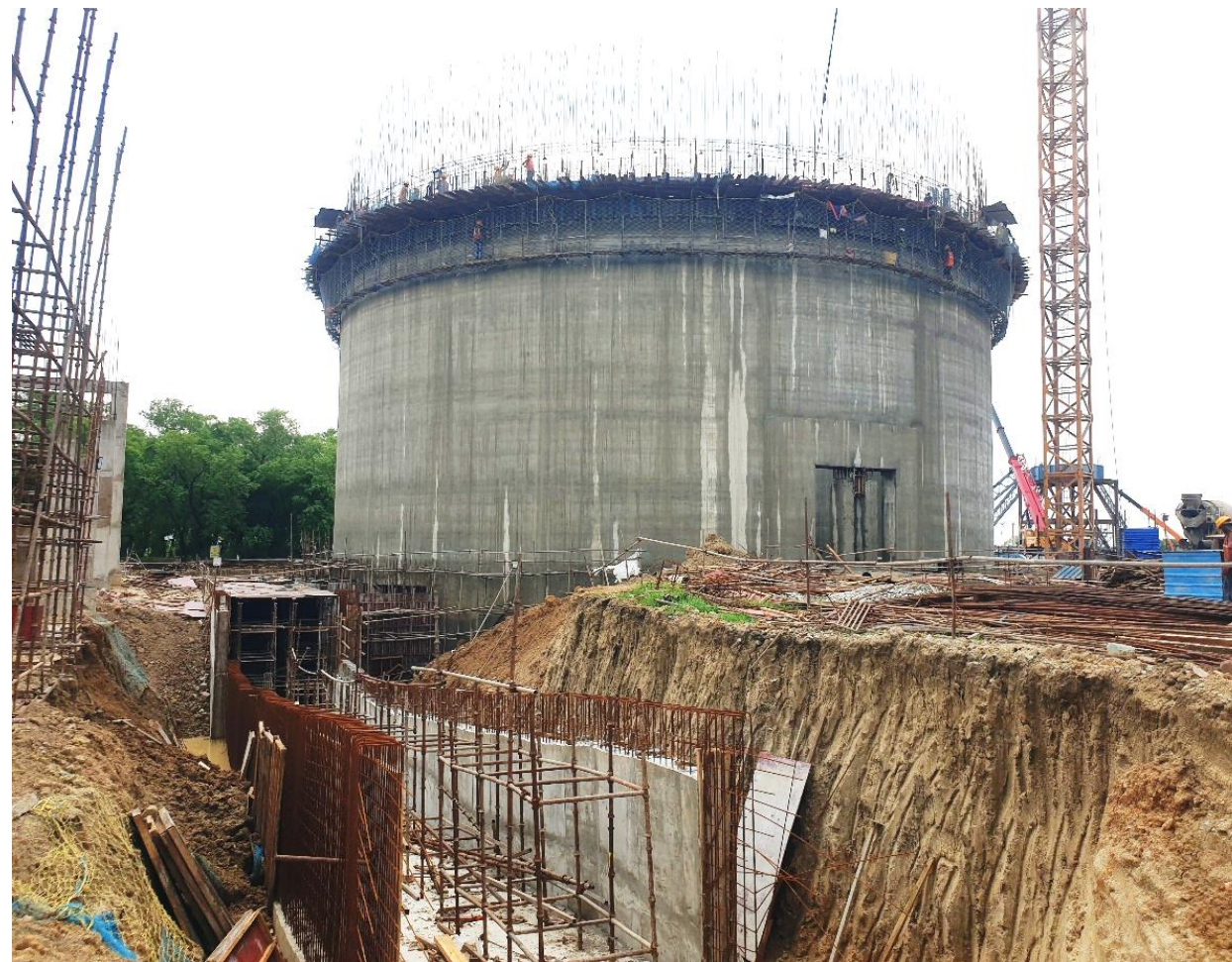
Clinker Silo & Cement Silo
