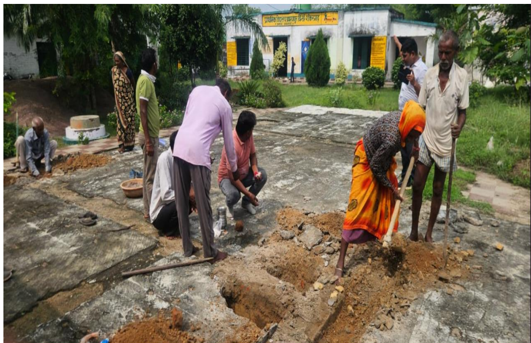
Renovation of Primary School
