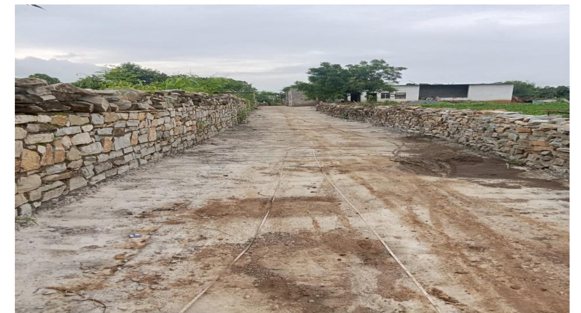
Construction of CC Road at village
