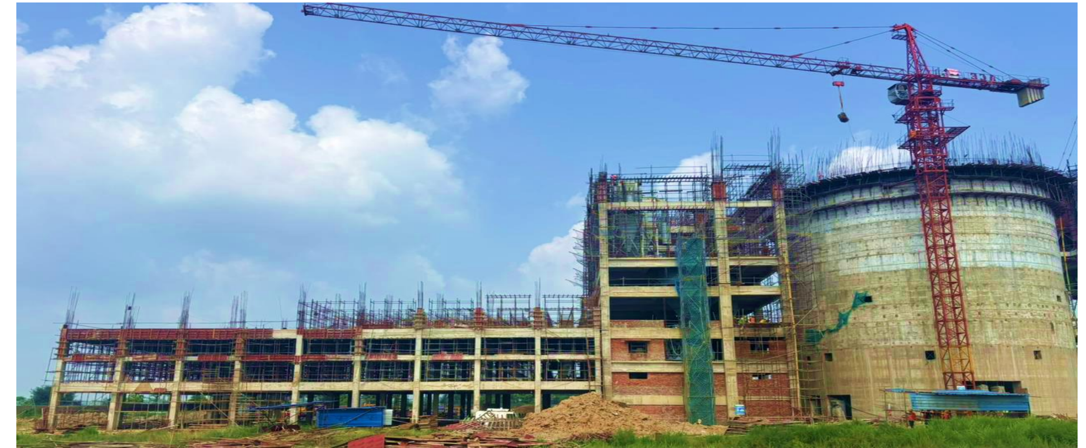
Packing Plant Building & Cement Silo
