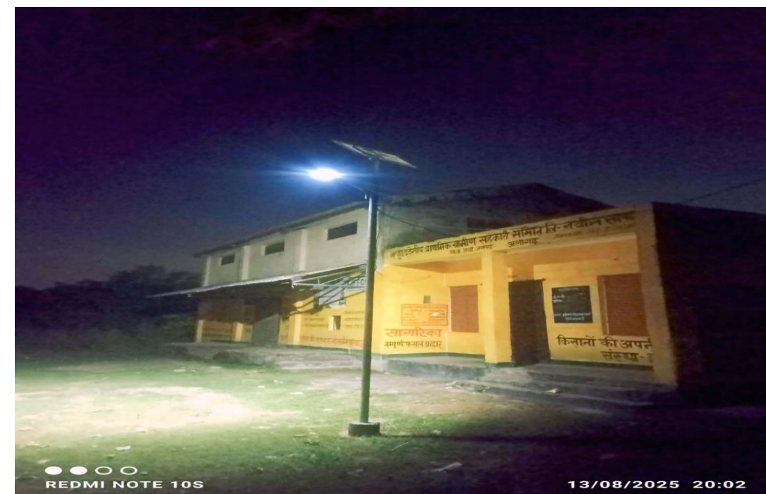
Solar Light Installation
