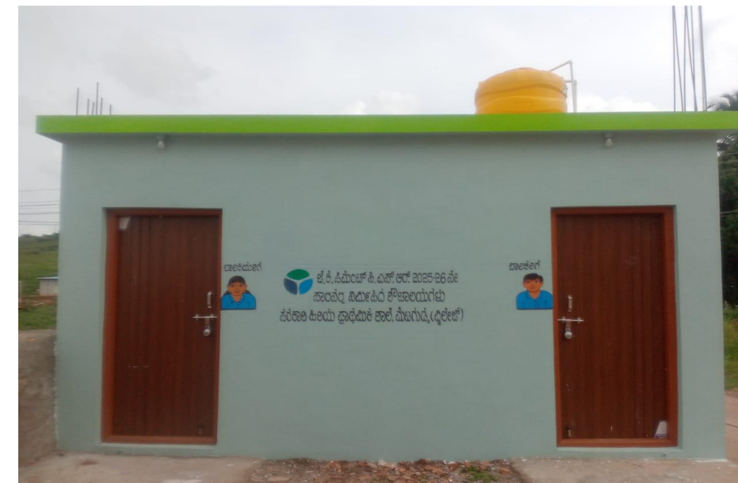
Construction of Toilet at School
