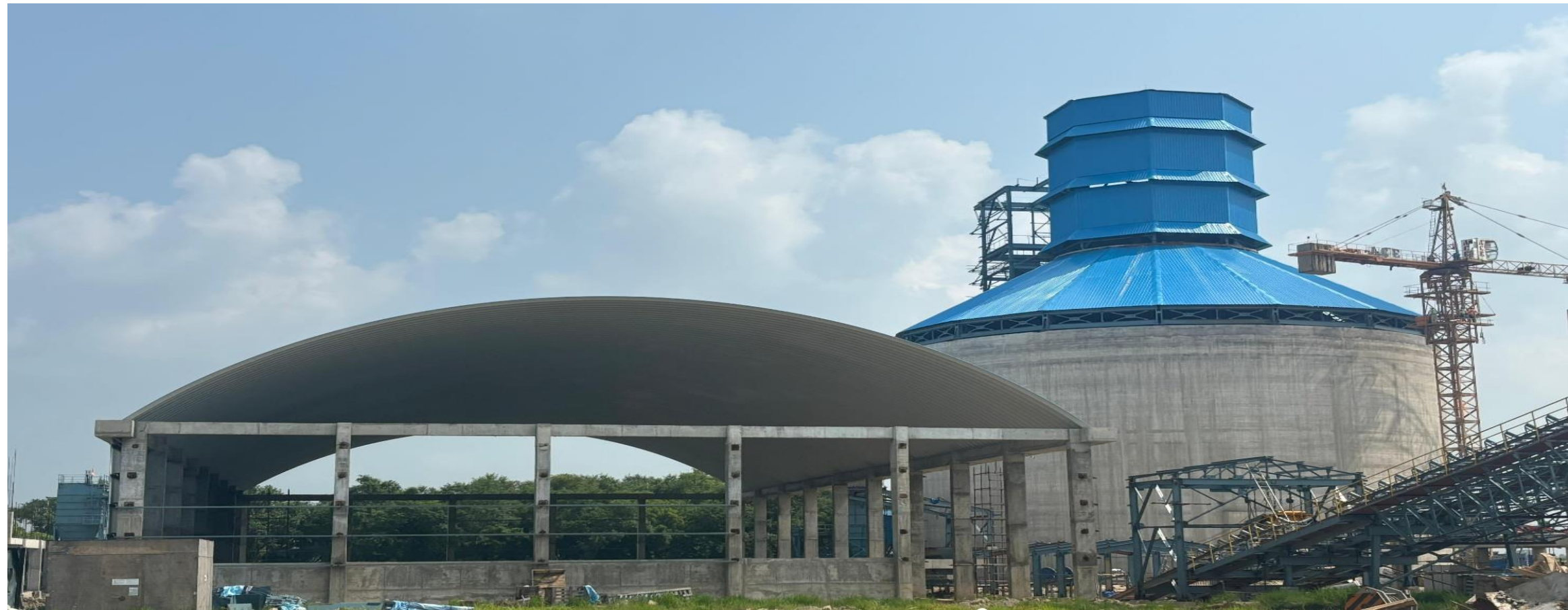
Additive Shed & Clinker Silo
