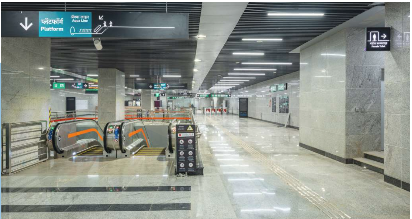
Environmental Control Systems (ECS) and Tunnel Ventilation (TVS) works at Mumbai Metro Line-3
