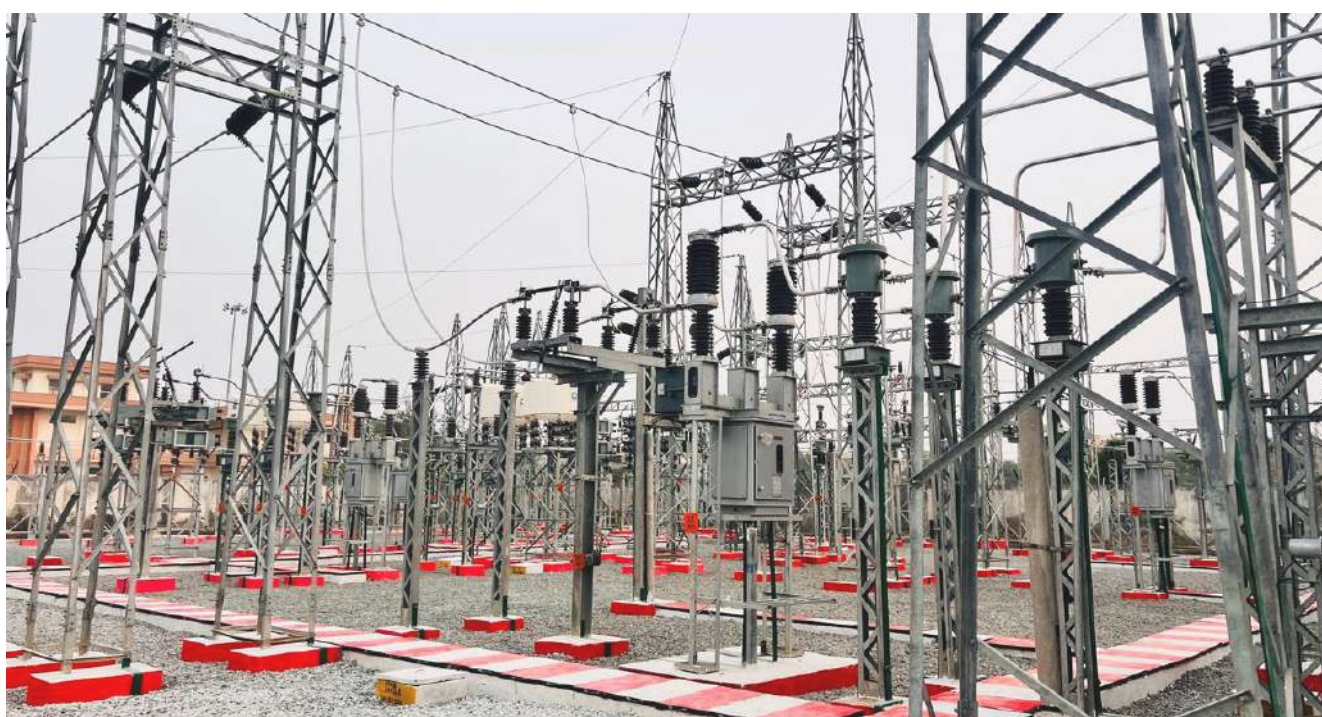
Railway Electrification: 2x25 kV Traction substation work at Gaya, Bihar
