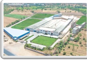
Amazone Dalpur Plant (Floor Tiles)
