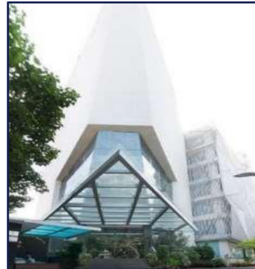
CCIL Bhavan Phase I : Upto 6 th floor
