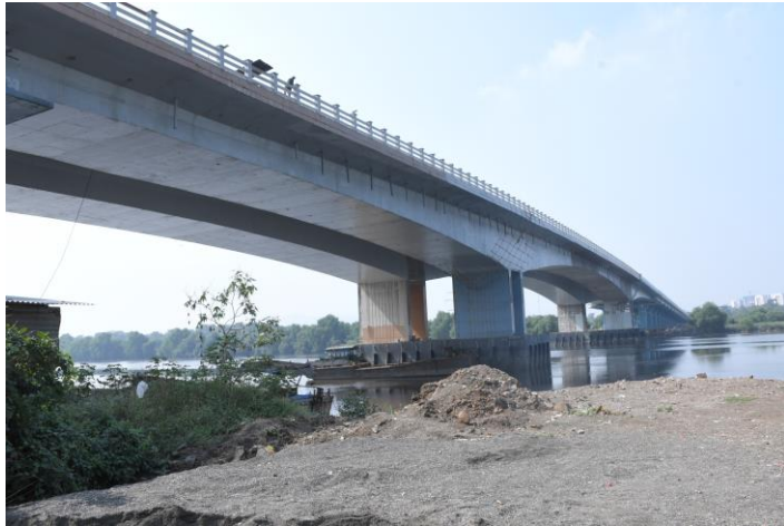
Motagaon Creek Bridge
