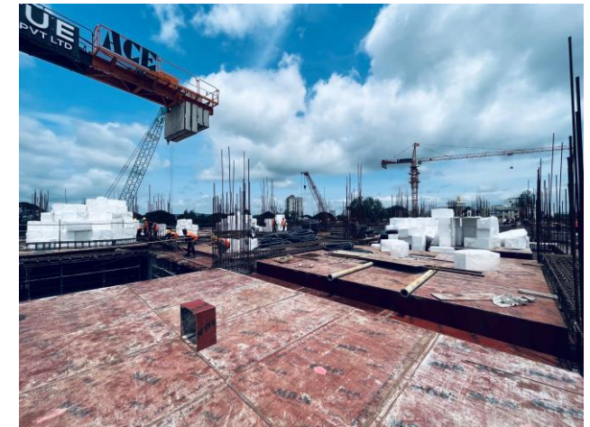
Pune Underground Metro
