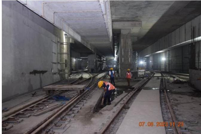
Mumbai Underground Metro Line 3
