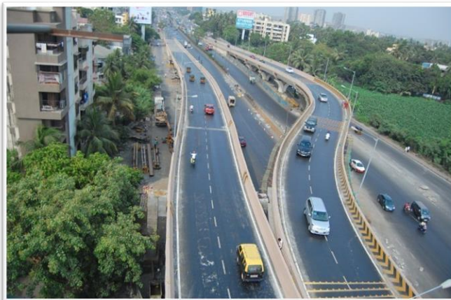
Amar Mahal Flyover
