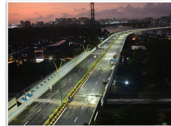
BKC- Chunabhatti Flyover
