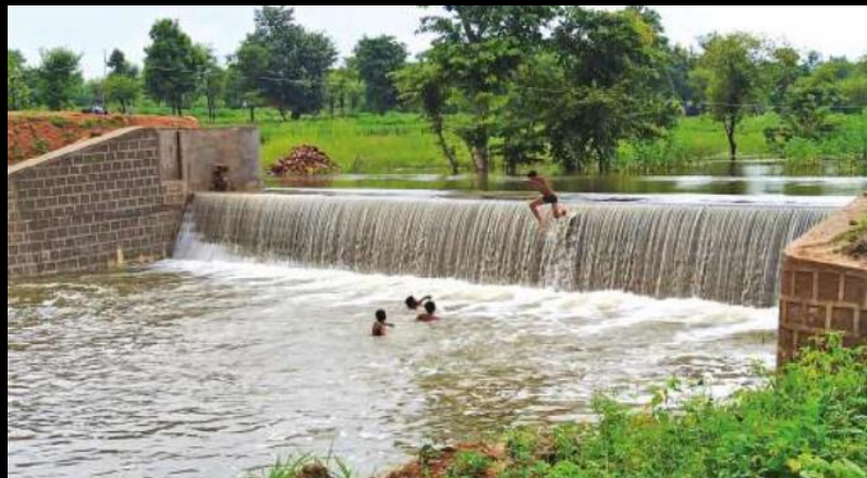
Recharging Ground Water Table
