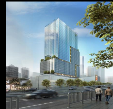
Project Rise, Lower Parel, Mumbai - ~1.10 msft
