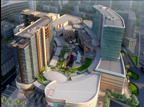
Phoenix MarketCity + Fountainhead Office Towers, Pune
