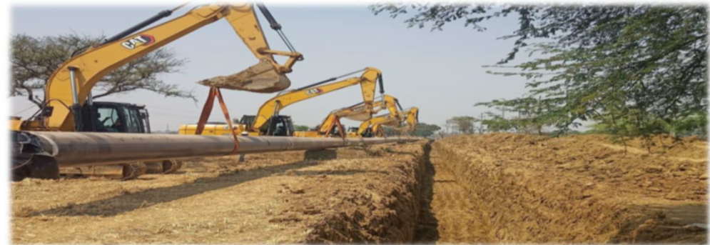
Setting up slurry pipeline
