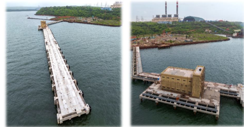
LPG construction at Jaigarh Port
