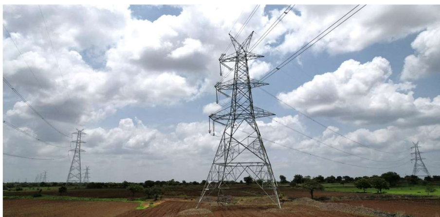
400kV Transmission line project in Solapur, Maharashtra
