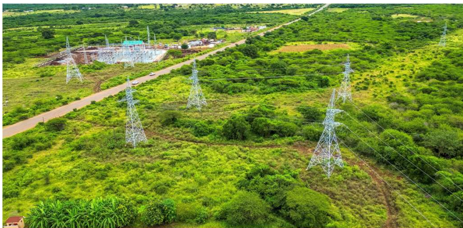
Eswatini 132kV Transmission Line Project
