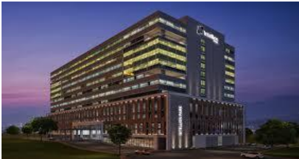
Intellion IT Park (Mumbai) SBA: 557k sf Capacity seats: ~14k
