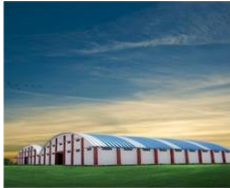
Roof with RCC Structure
