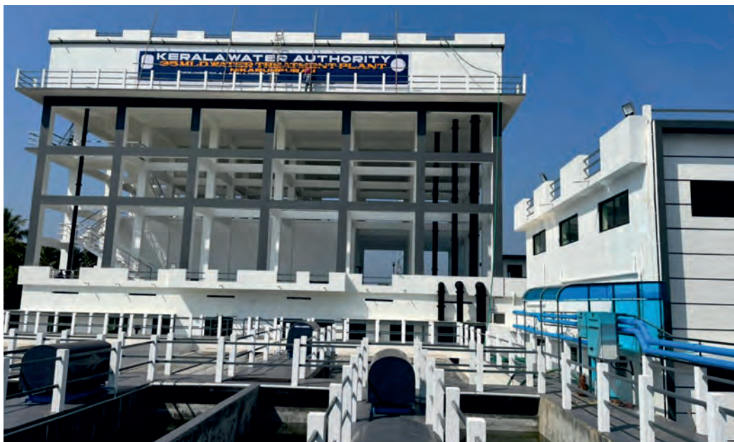
Water Treatment Plant at Chengannur Municipality, Kerala
