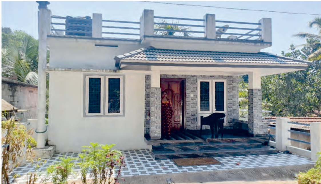
Construction of Houses for EWS (Urban), Kerala
