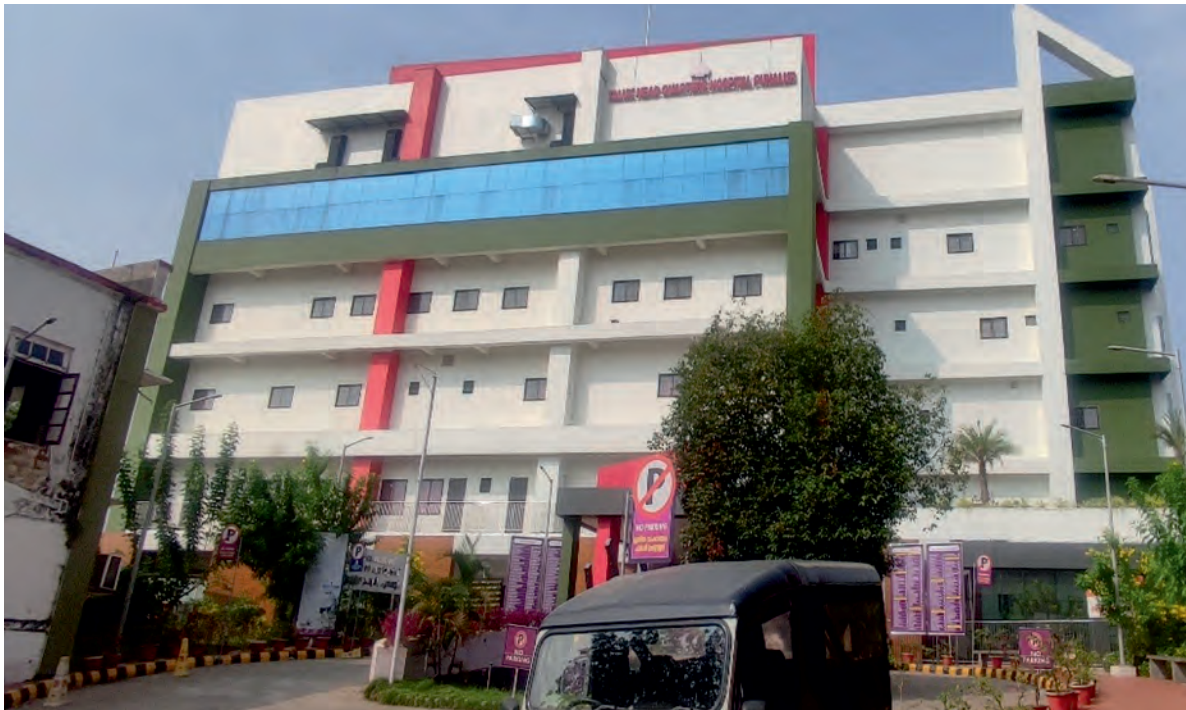
Taluk Head Quarters Hospital, Punalur, Kollam District, Kerala
