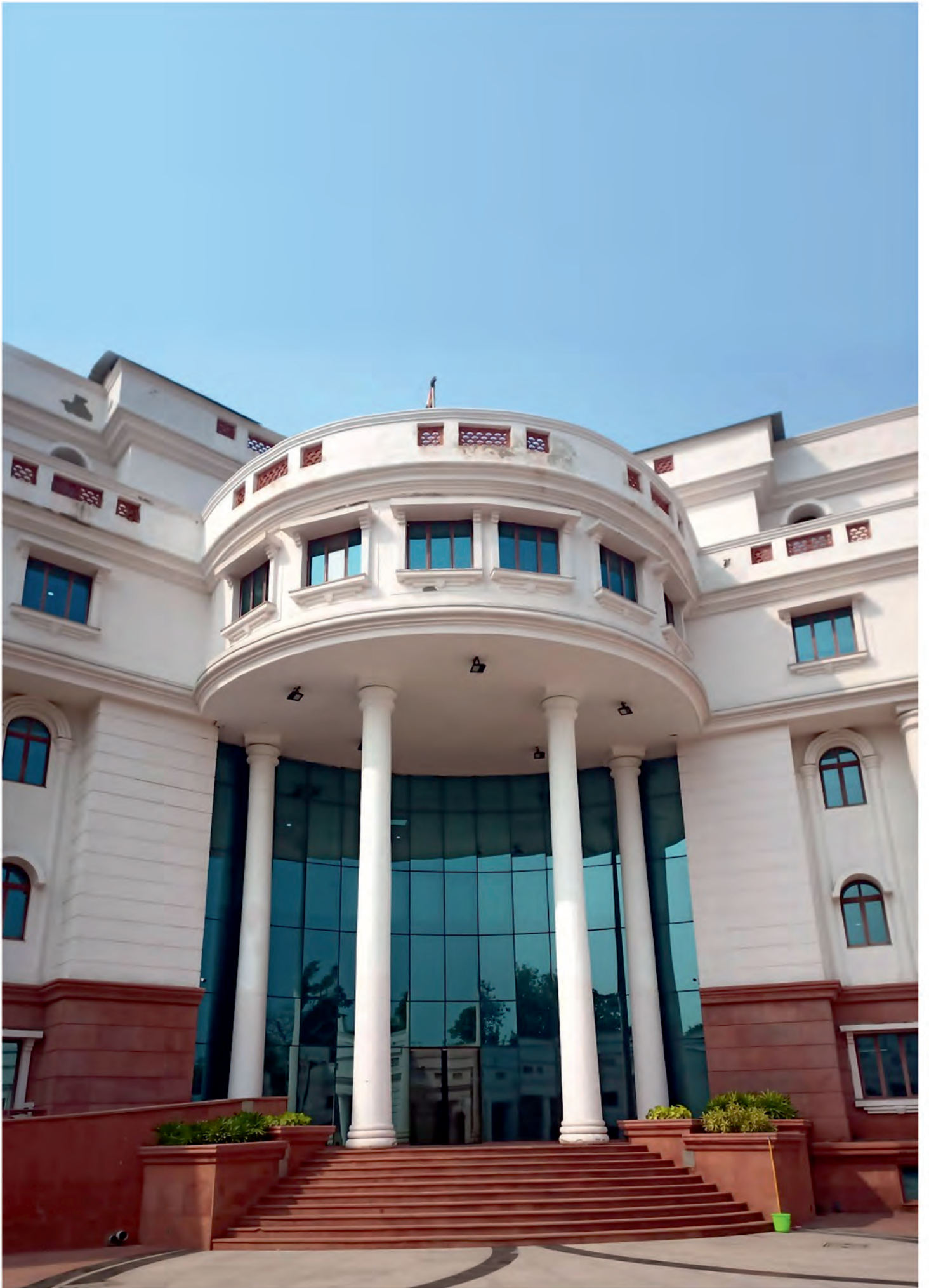
Office Building for Archeological Survey of India, New Delhi
