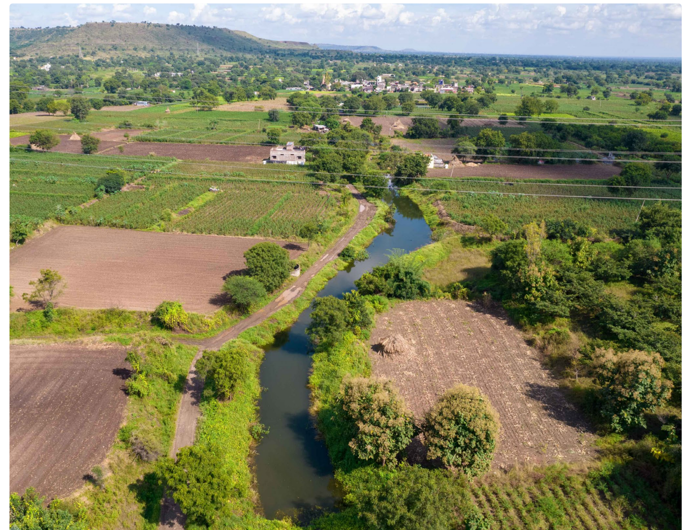
Canal deepened to increase water capacity
