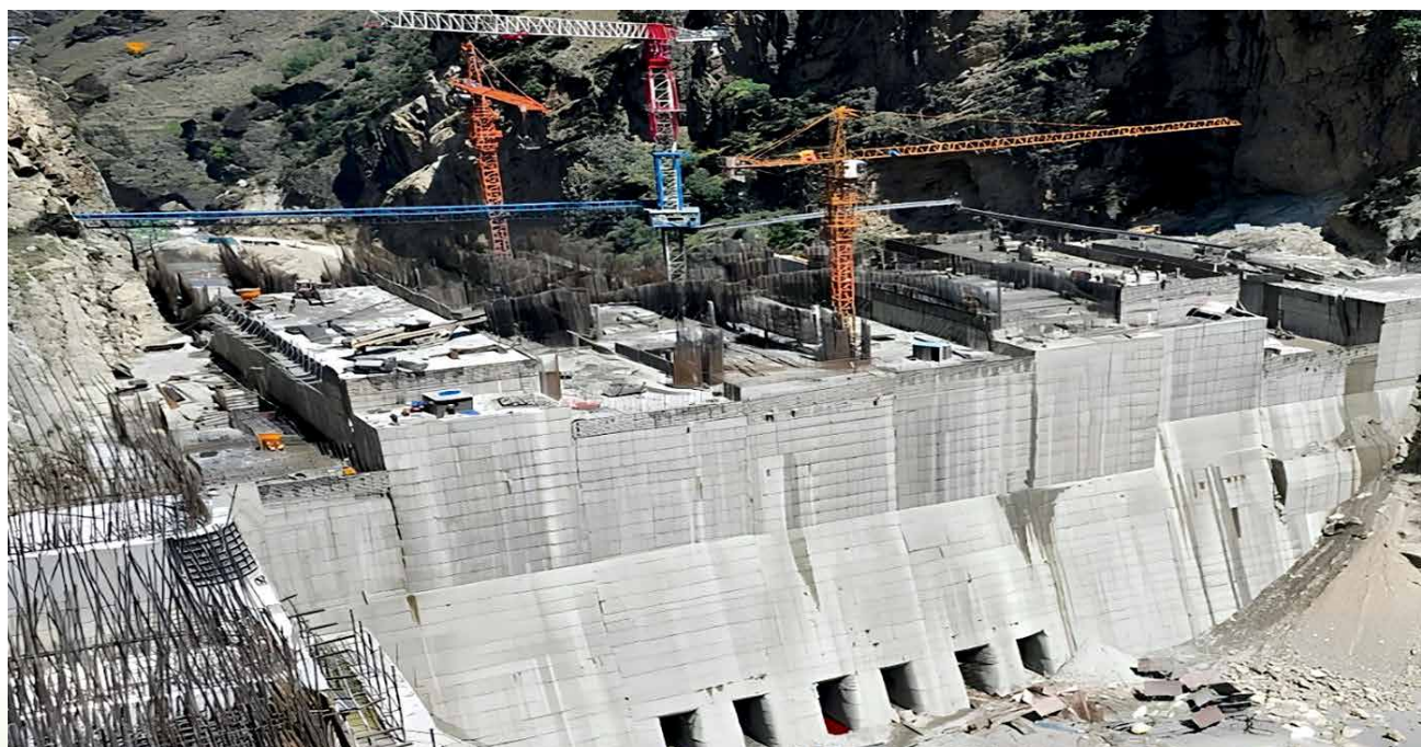
CONCRETING OF DAM – 624 MW KIRU PROJECT (UT OF J&K)
