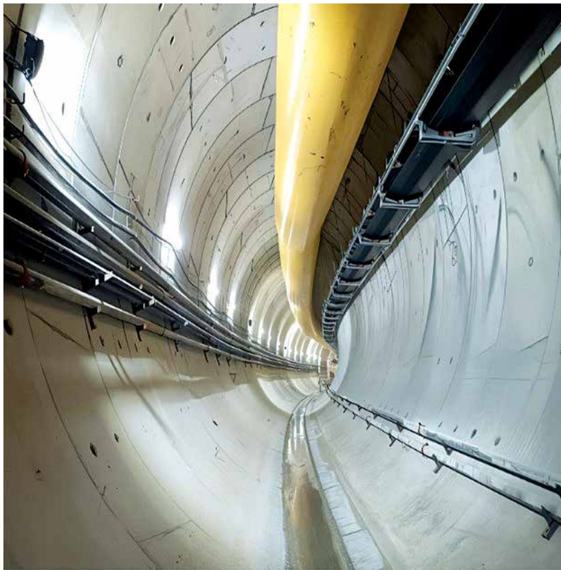
HRT-2 by TBM– 1000 MW PAKALDUL PROJECT (UT OF J&K)
