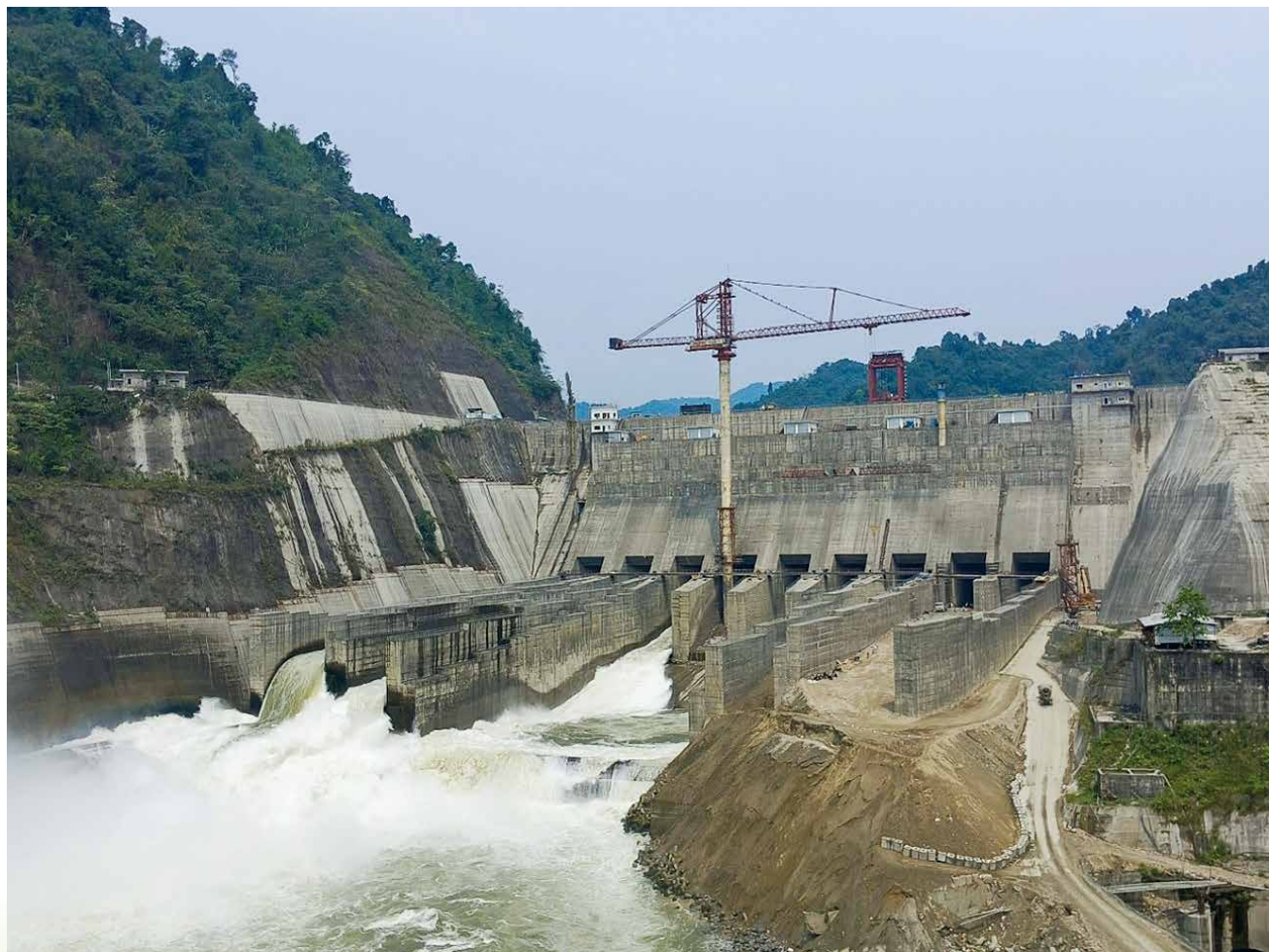
116 M HIGH CONCRETE GRAVITY DAM (DOWNSTREAM VIEW) – 2000 MW SUBANSIRI LOWER PROJECT (ARUNACHAL PRADESH)
