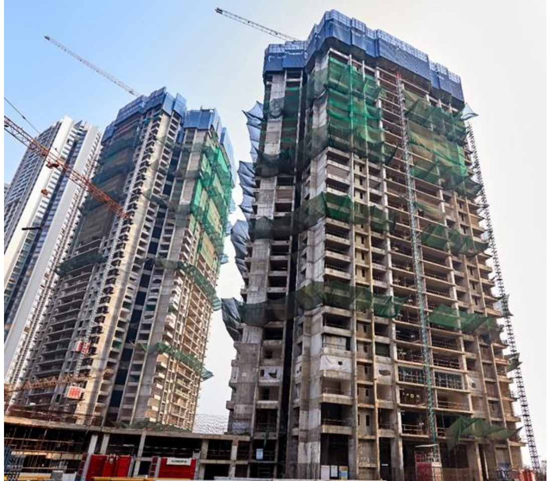
Project status as on Dec 31, 2023
