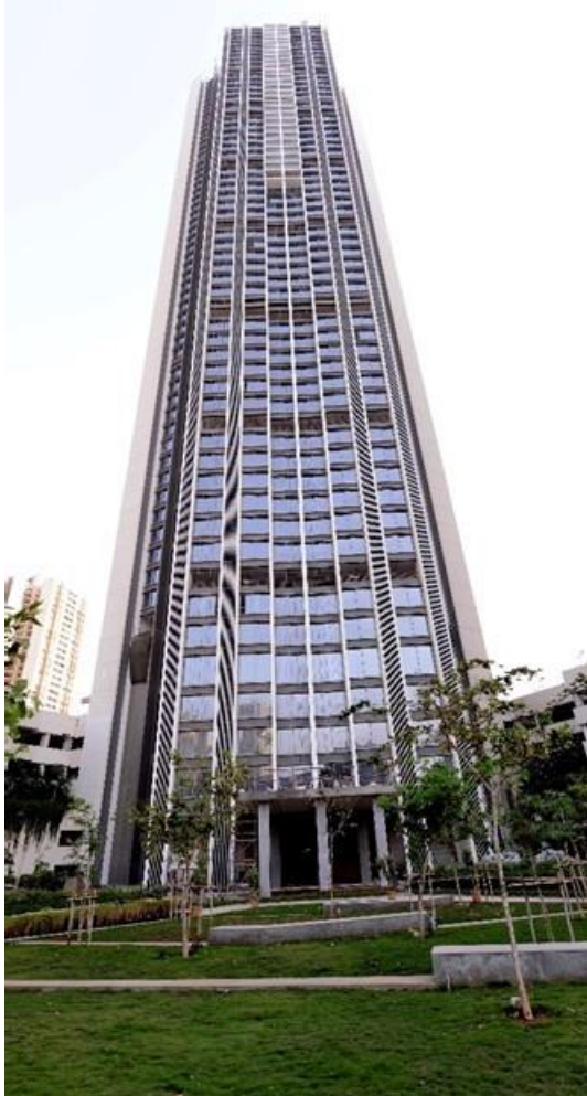
Project status as on Mar 31, 2022
