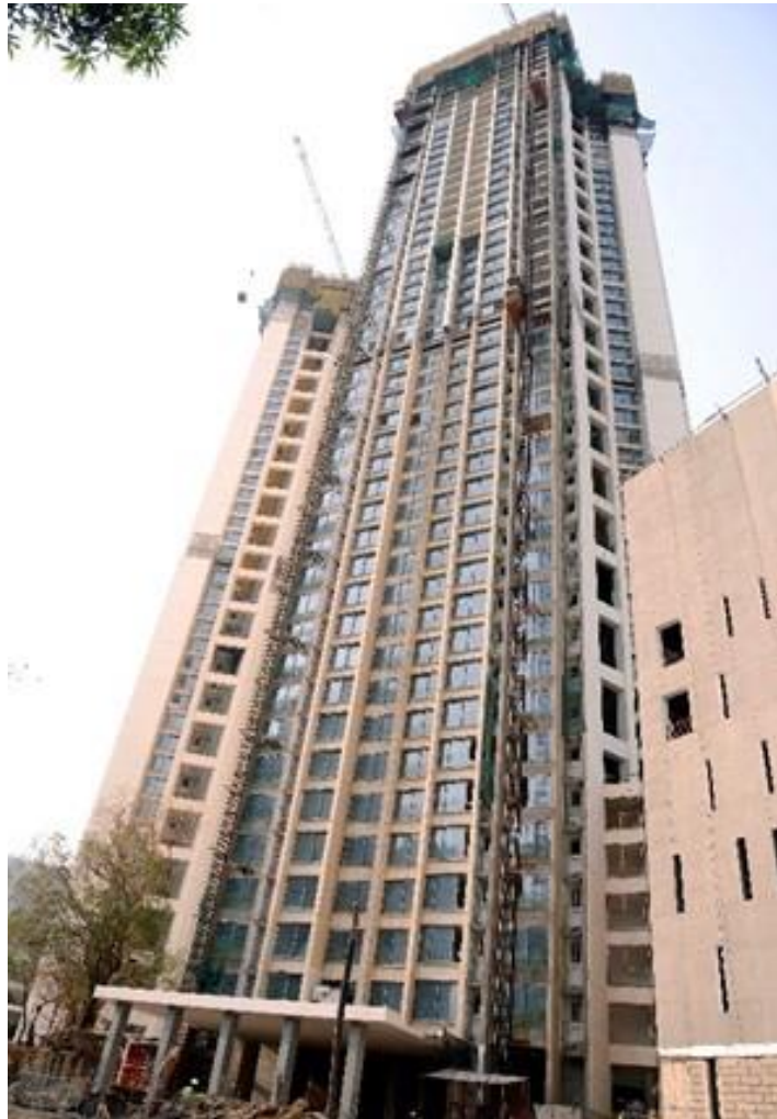
Project status as on Mar 31, 2022
