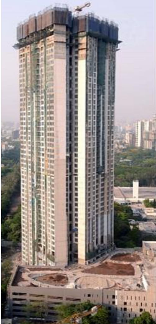
Project status as on Mar 31, 2022
