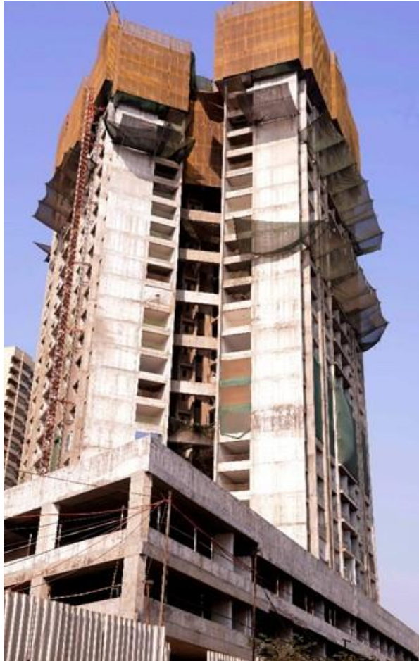
Project status as on Mar 31, 2022
