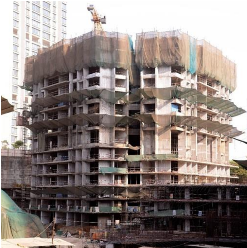
Project status as on Mar 31, 2022
