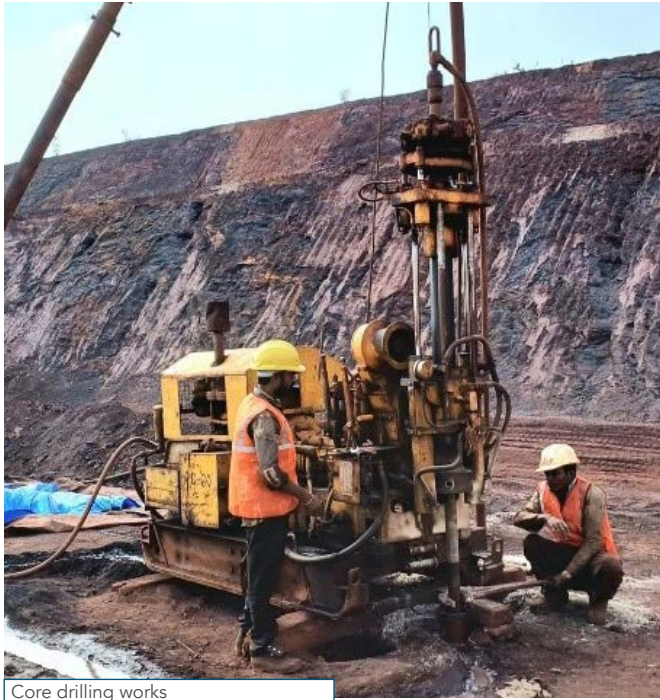
Core drilling works
