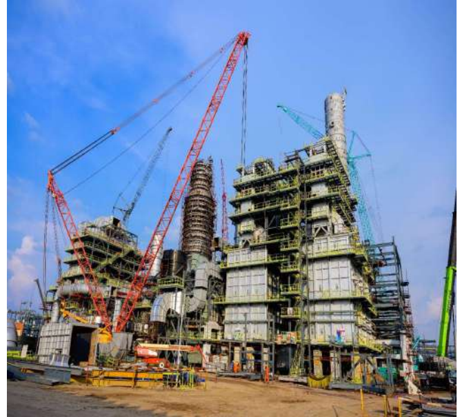
HRRL Project, Rajasthan
