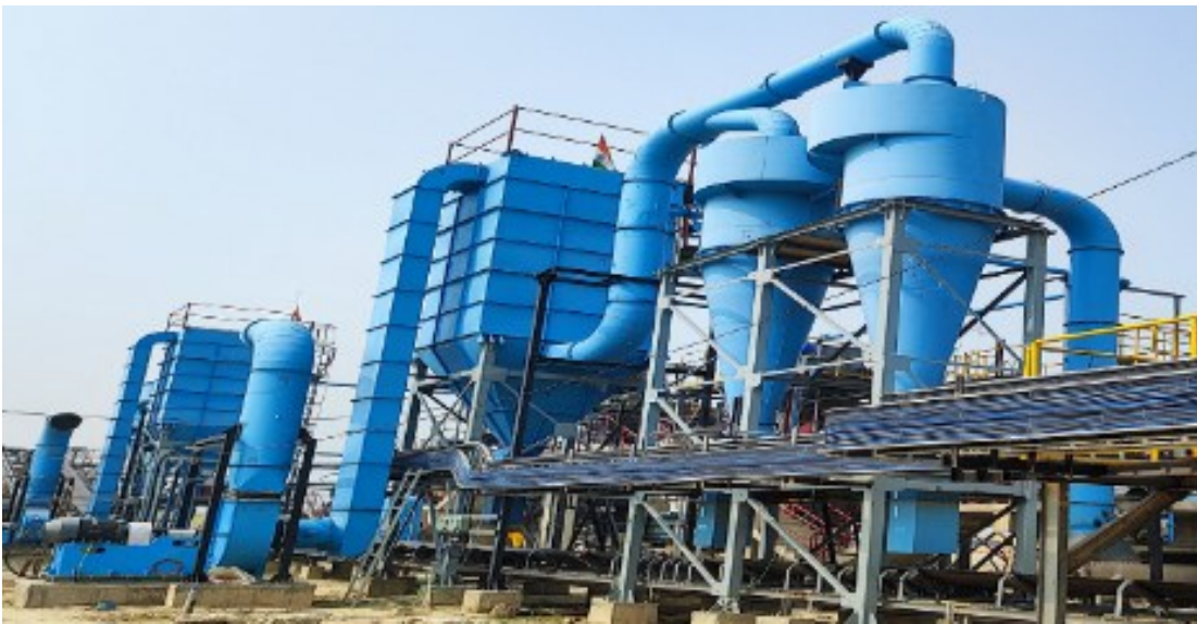
CBG Plant at Budaun- Milling Section
