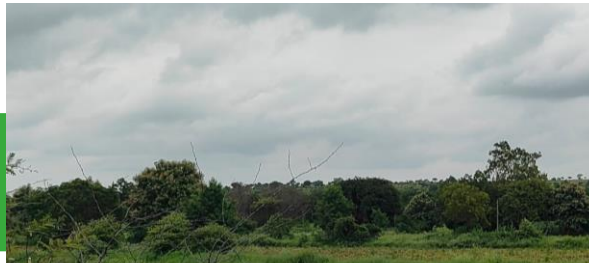
131 MWp Ground Mounted project at Nashik, Maharashtra
