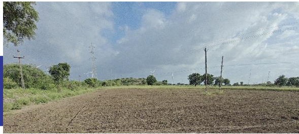
105 MWp Ground Mounted project at Jamnagar, Gujarat
