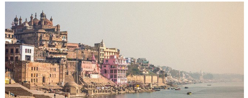
Continuous emission monitoring for Varanasi municipality project
