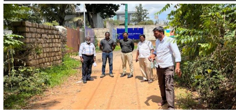
Phase-2 Nelamangala rural road development project initiated
