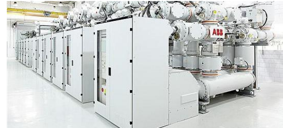
Gas insulated switchgear for an energy company
