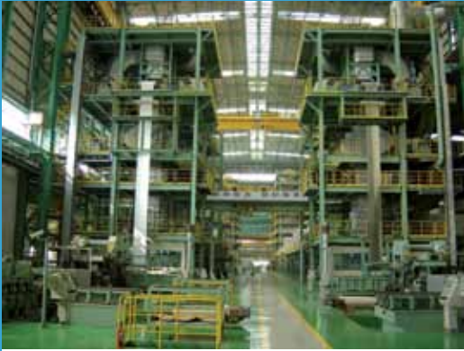
Continuous Galvanizing Line
