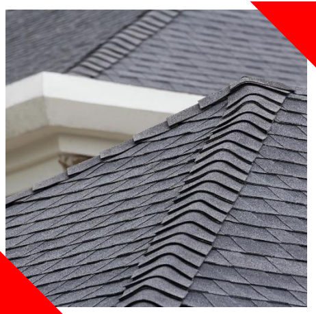
Fibre Cement Roof
