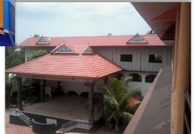
Roof Top Extension - (V-Panel )
