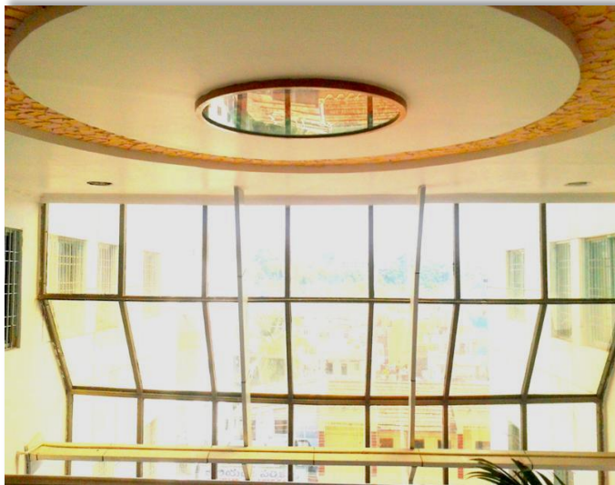
Concealed Grid False Ceiling - (V-Board/V-Designer)
