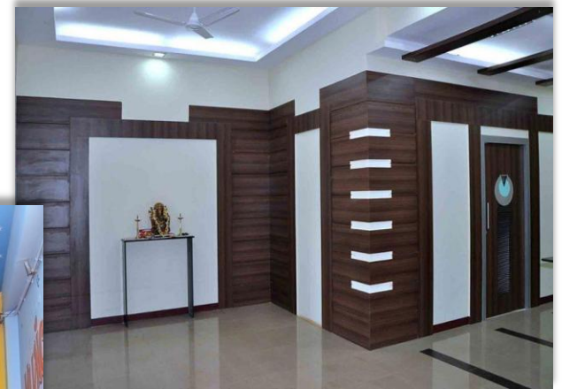
Internal partition - (V-Panel)
