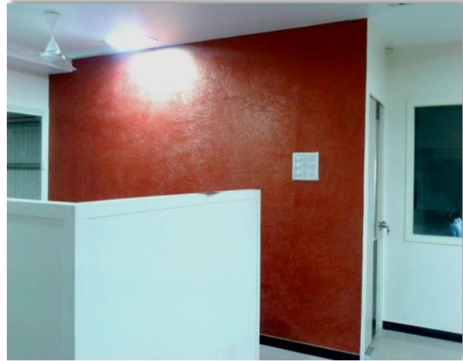
Wall Paneling - (V-Board)
