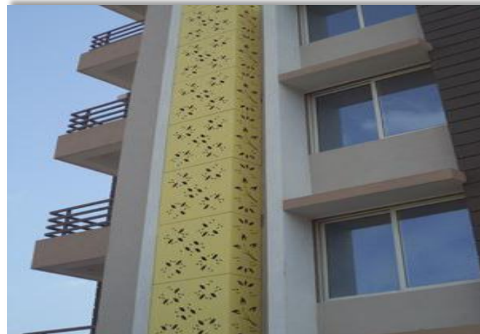
Duct Covering - (V-Board - Premium)
