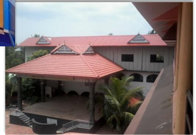
Roof Top Extension - (V-Panel )
