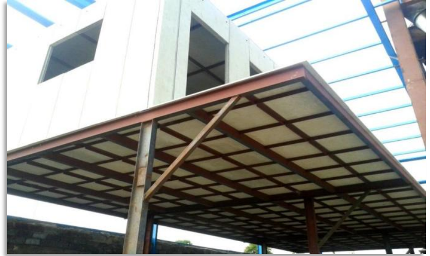
Mezzanine flooring - (V-Board)
