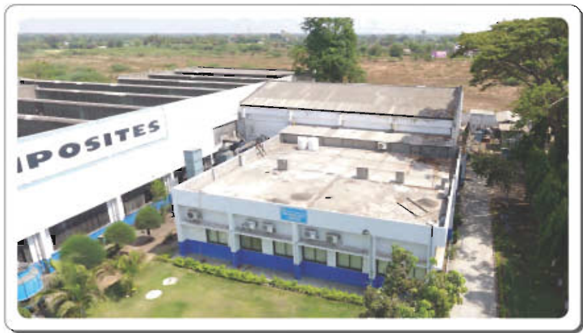
Technology center at Paithan
