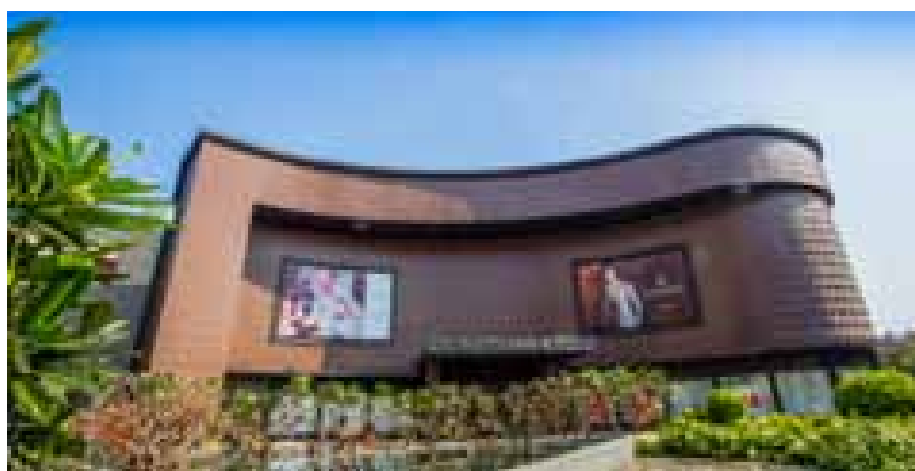
Palladium Mall Exterior (Actual Image)
