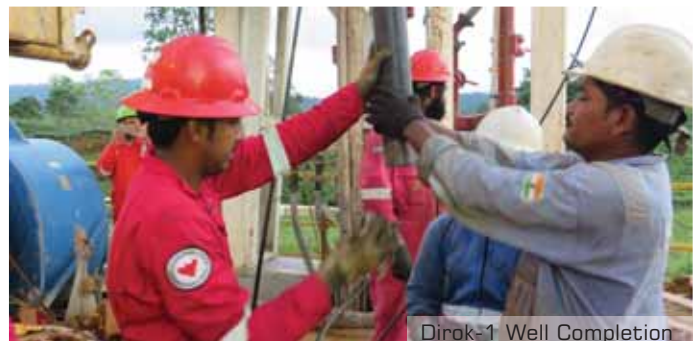
Dirok-1 Well Completion
