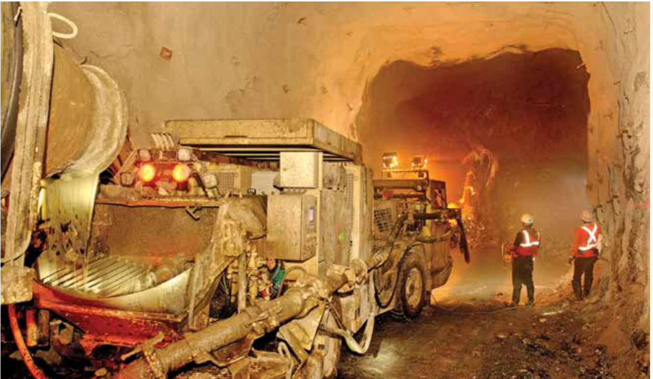
○ Shotcreting operation at Rampura Agucha Underground mine
