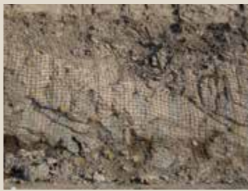
A typical cable bolting-cum-wire meshing site at Rampura Agucha open cast
