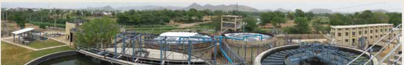
○ Sewage Treatment Plant in Udaipur
