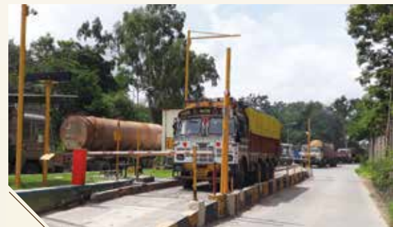
Technology upgradation: Man-less weigh bridge
