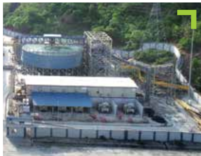
Dry Tailing Plant
