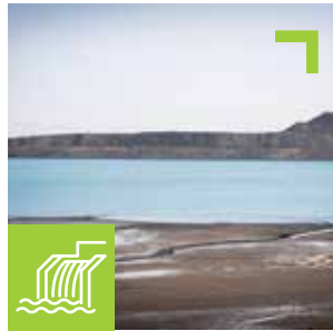
TAILINGS DAMS MANAGEMENT
