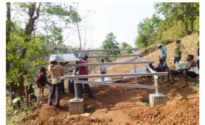
Solar panel installation for water lifting
