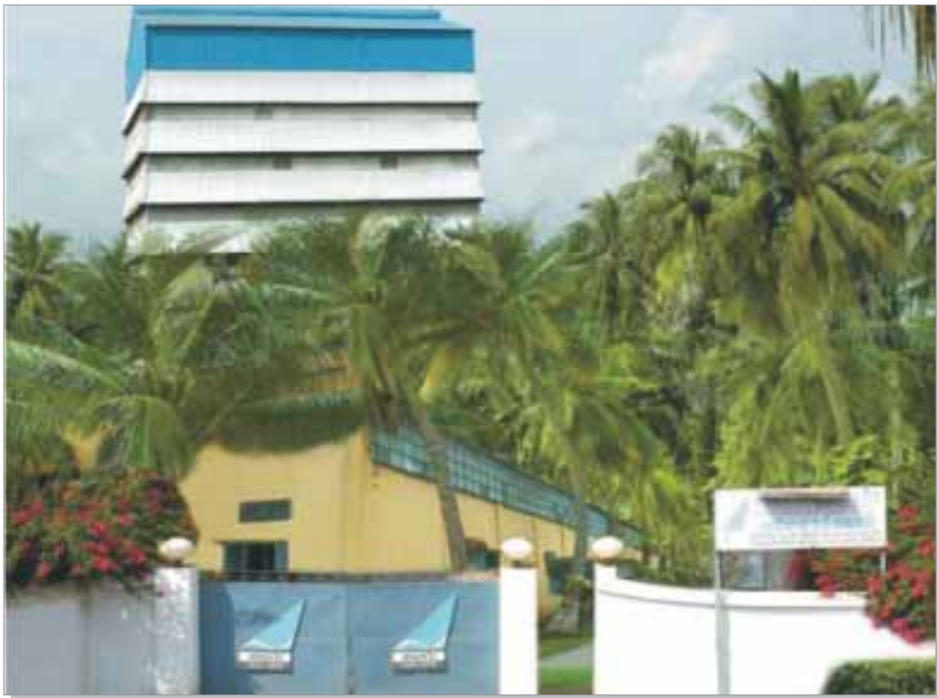
Shrimp Feed Plant located at Kovvur, West Godavari District, Andhra Pradesh
