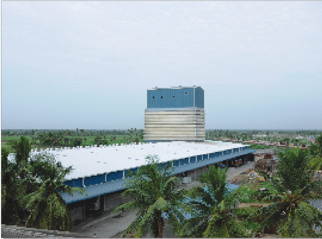
New shrimp feed manufacturing plant at Kovvur
