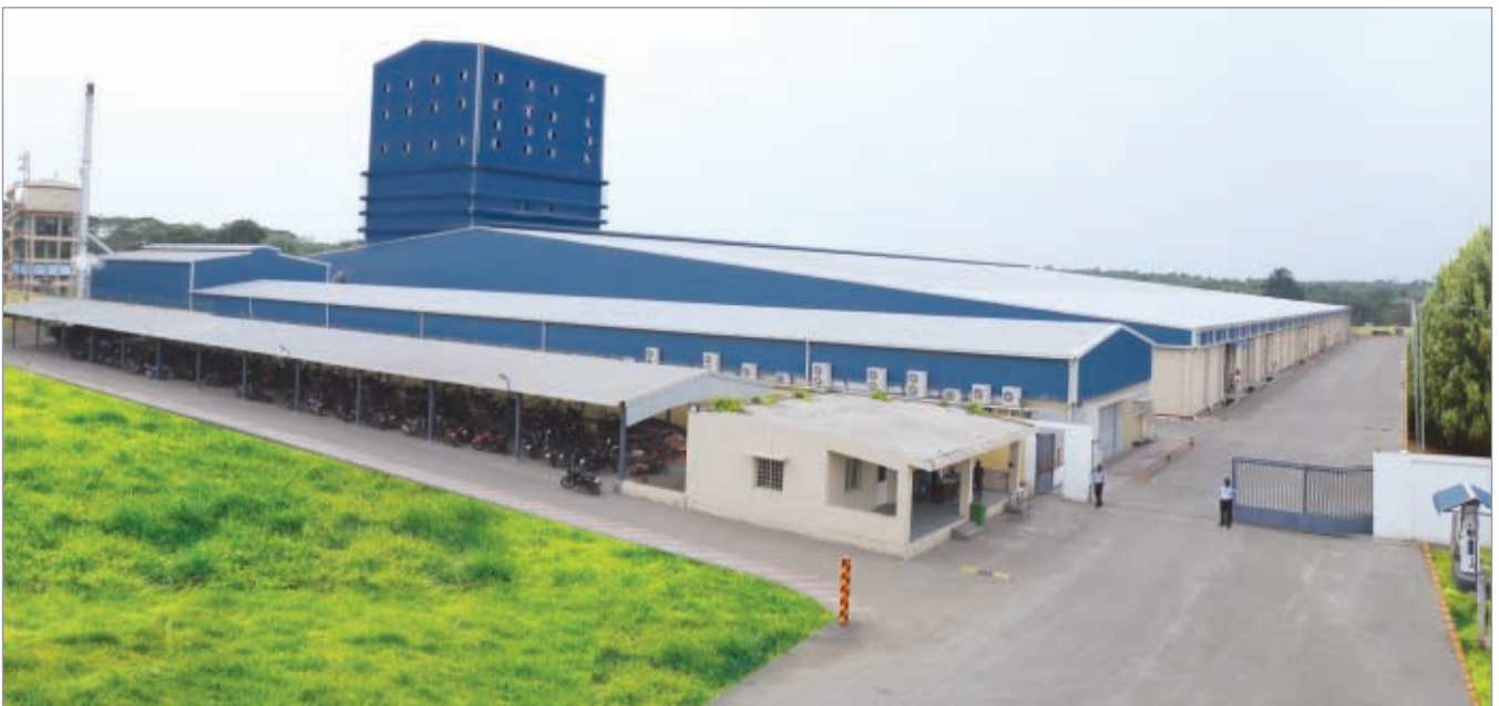
New shrimp feed plant at Bandapuram.
