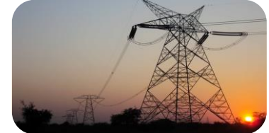
Longest Private HDVC Line in India
