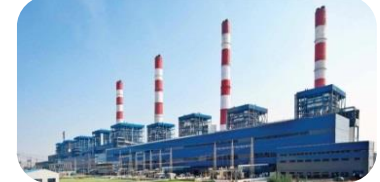
Largest Private Thermal Power Station in India
